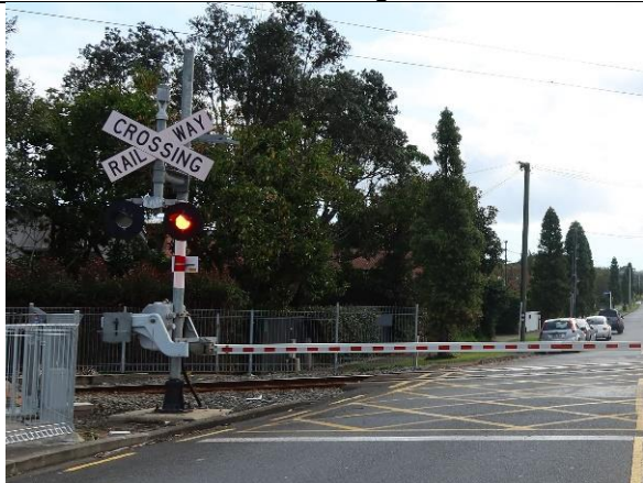
View of signalling when crossing is activated on the correct side of the road
