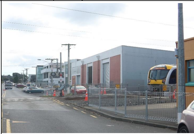
View of signalling when crossing is activated on the wrong side of the road (half-arm barrier has very low visibility and flashing lights are not observable)
