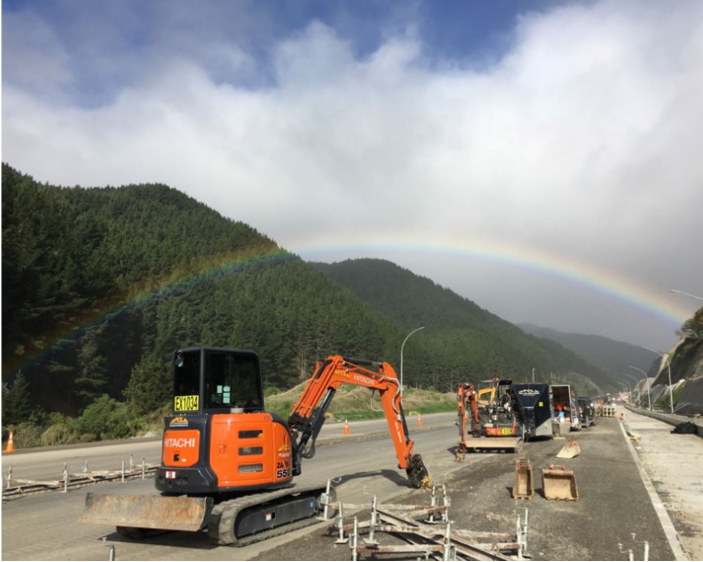
Transmission Gully Channel Drains– PCL Contracting
