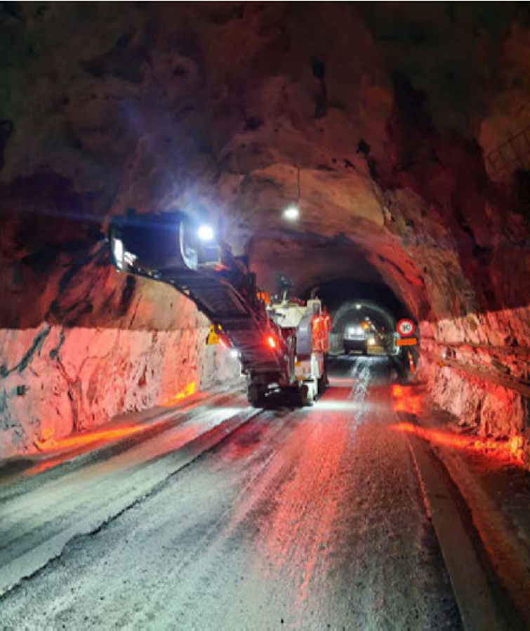
Homer Tunnel Resurfacing Works - Downer NZ
