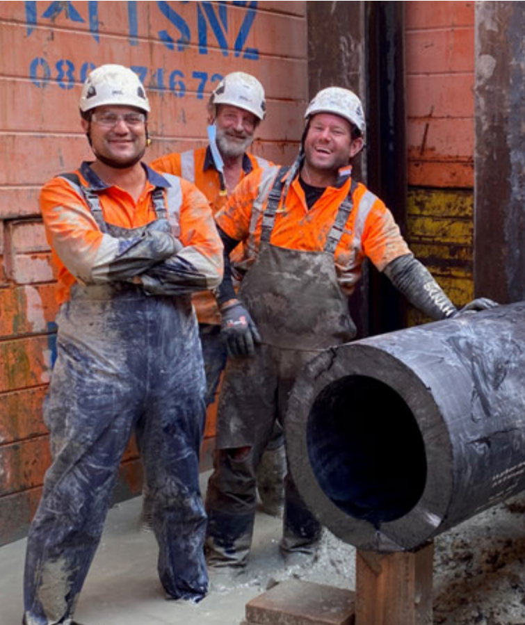
City Rail Link Wastewater Diversion – Universal Underground
