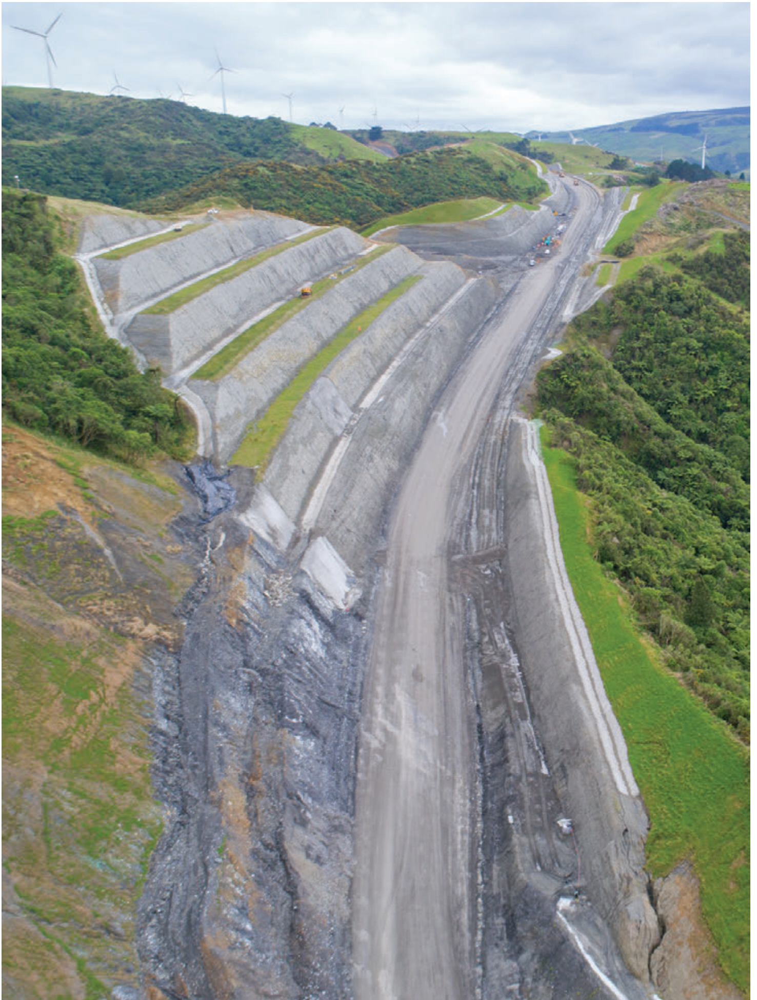
11.5 kilometre Manawatū to Tararua Highway (SH3) – HEB Construction
