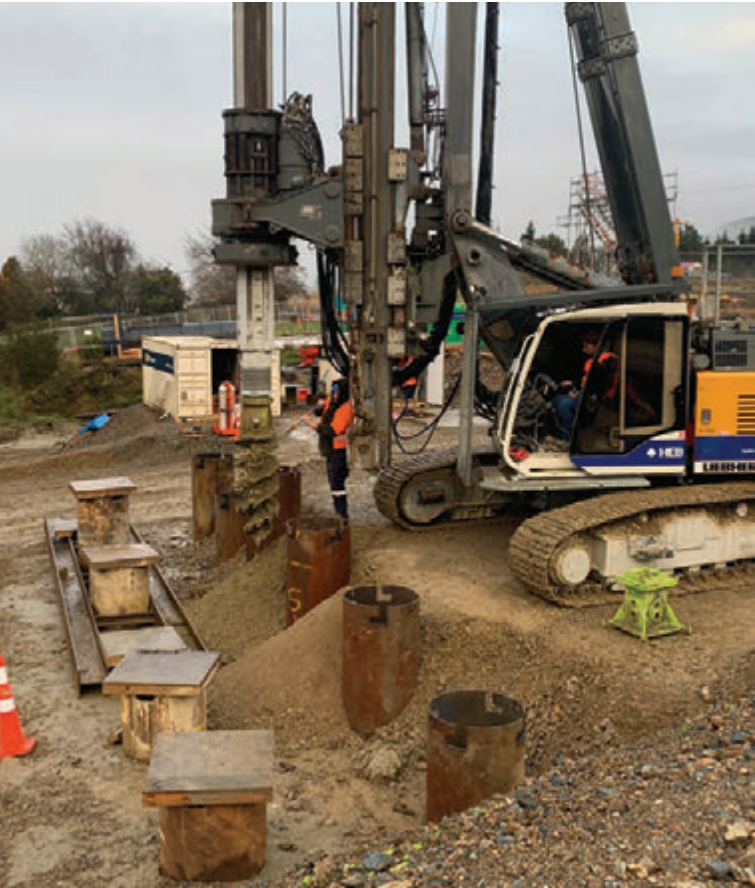
Drilling pile foundations for an abutment for the Clutha River bridge at Beaumont – HEB Construction
