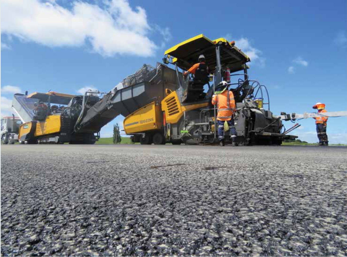
Asphalting the Waikato Expressway.
