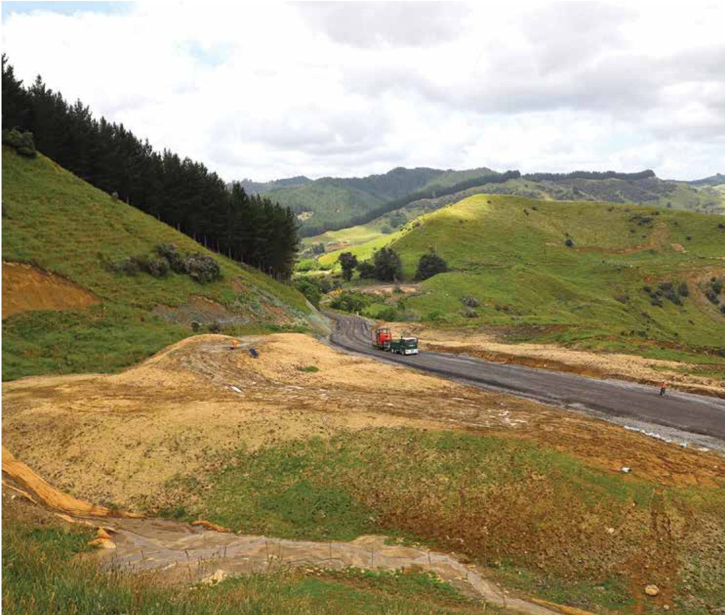
Whanganui - Raetihi SH4 repairs underway.
