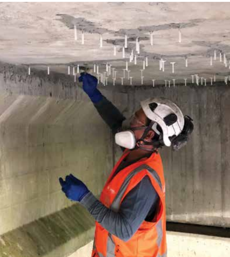
SH2 Waioeka Gorge Bridge Strengthening.
