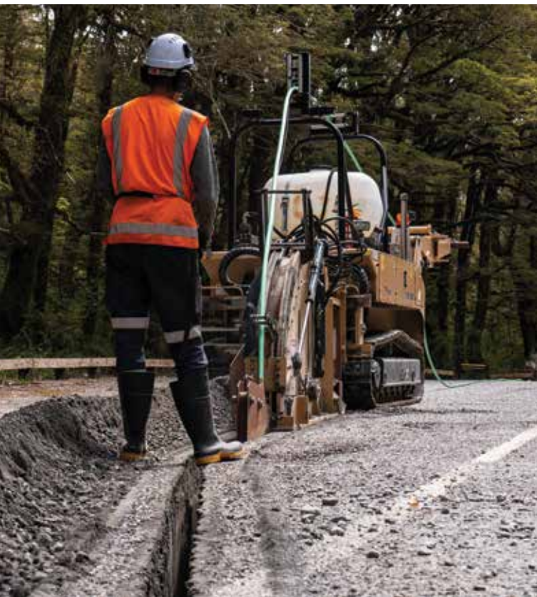
Optic fibre cable laying between Haast and Lake Hawea – Marais Laying.
