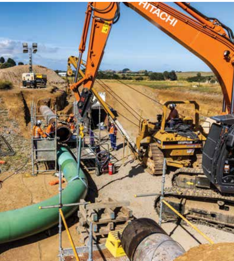
Maui Gas pipeline realignment.
