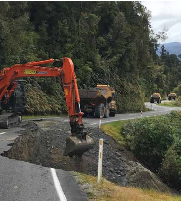
MBD Contracting working on slip repairs, West Coast.
