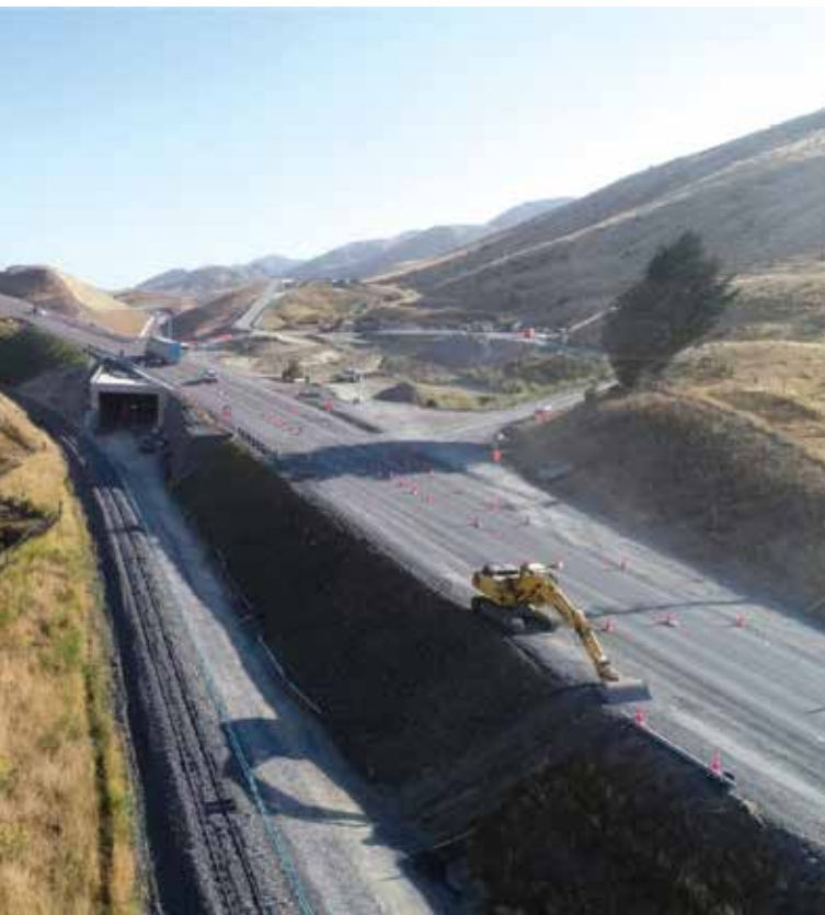
Tar Barrel Tunnel Bypass – HEB Construction.
