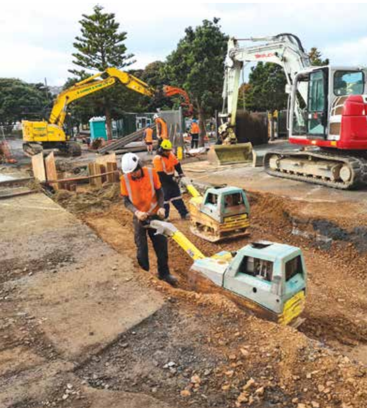
Jervois Quay stormwater replacements – E Carson & Sons.
