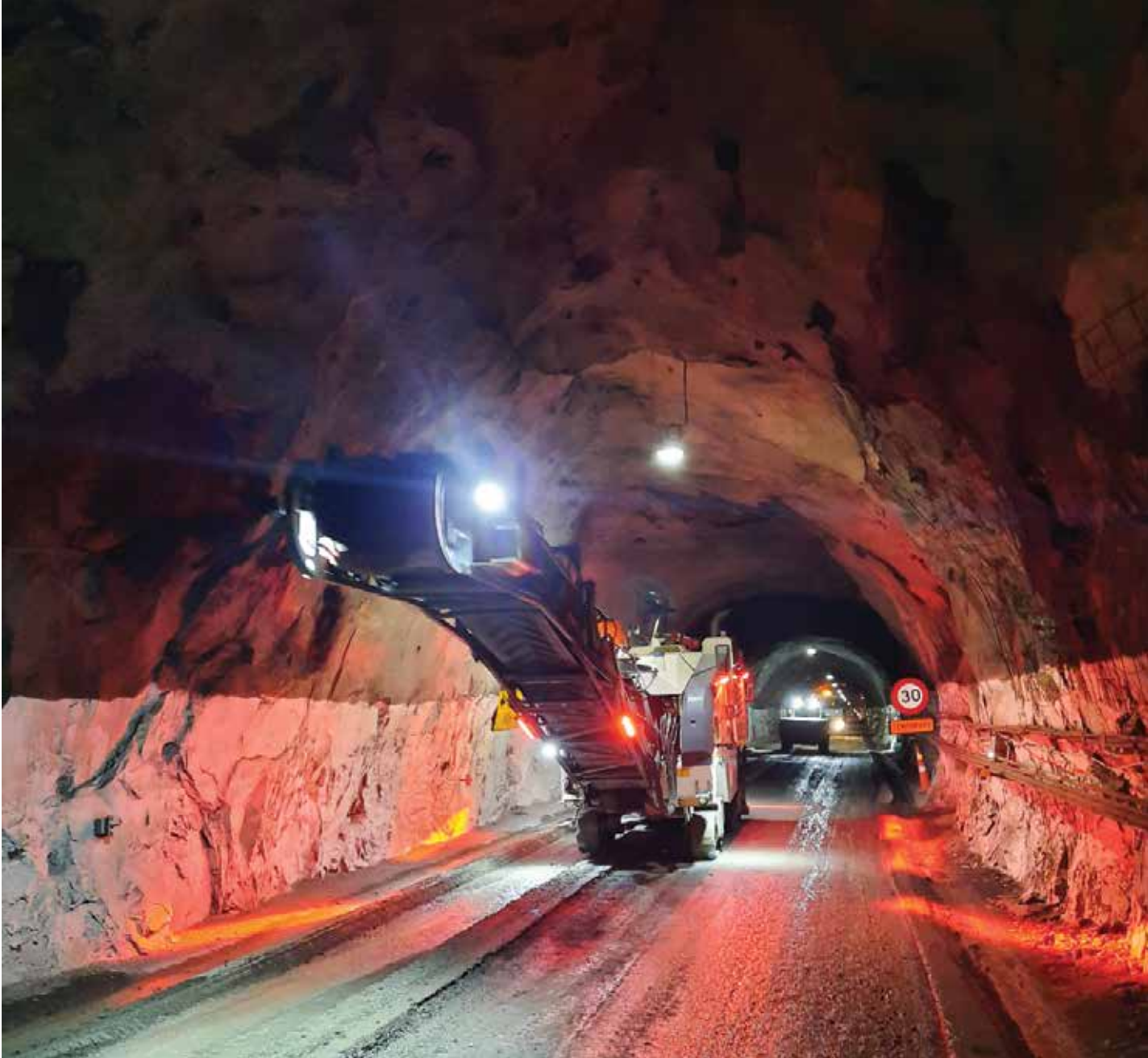
Homer Tunnel resurfacing works – Downer NZ.
