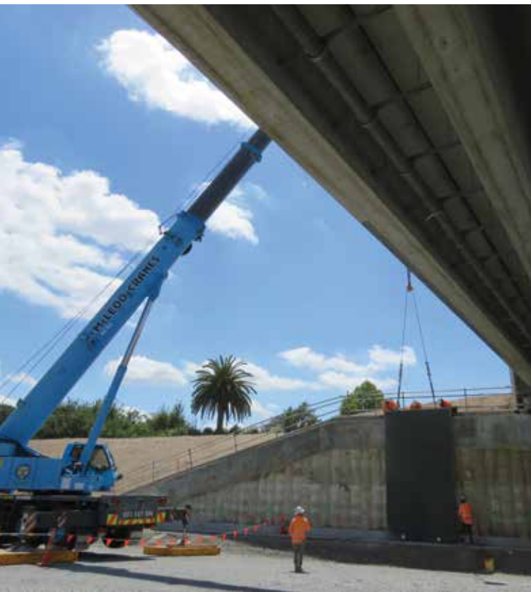
Placing panels on the Waikato Expressway.
