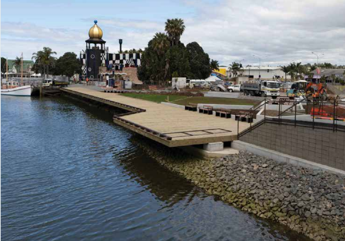
Civil and landscaping works at the Hundertwasser Art Centre – Robinson Asphalts.
