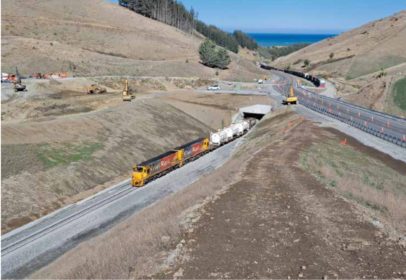
The new Ruakanakana Underpass – HEB Construction.
