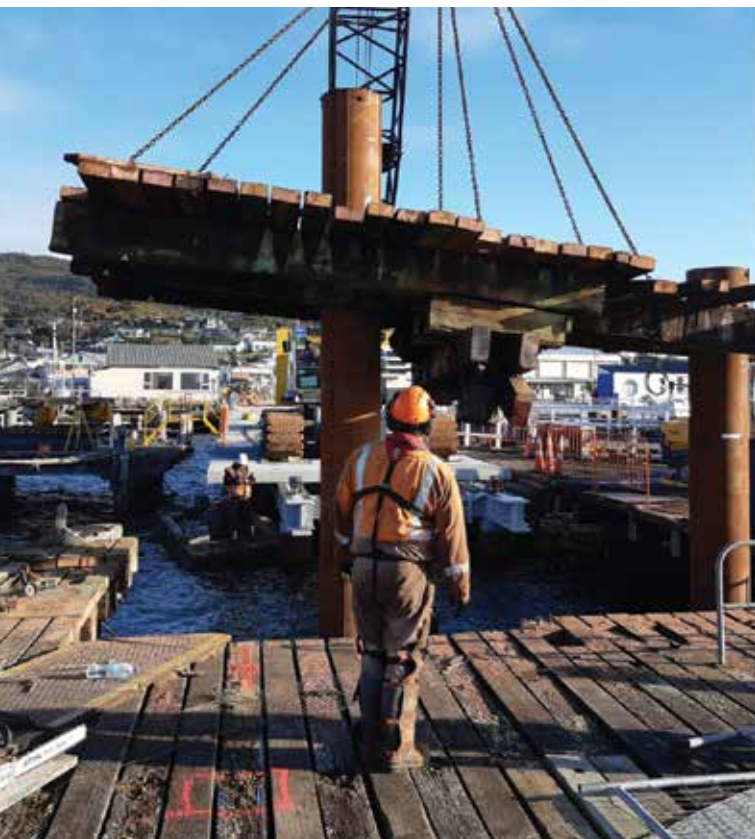
Bluff Town Wharf upgrade – Brian Perry Civil.
