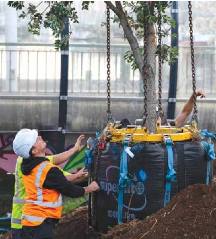
Hundertwasser Art Centre, transplanting – Robinson Asphalts.
