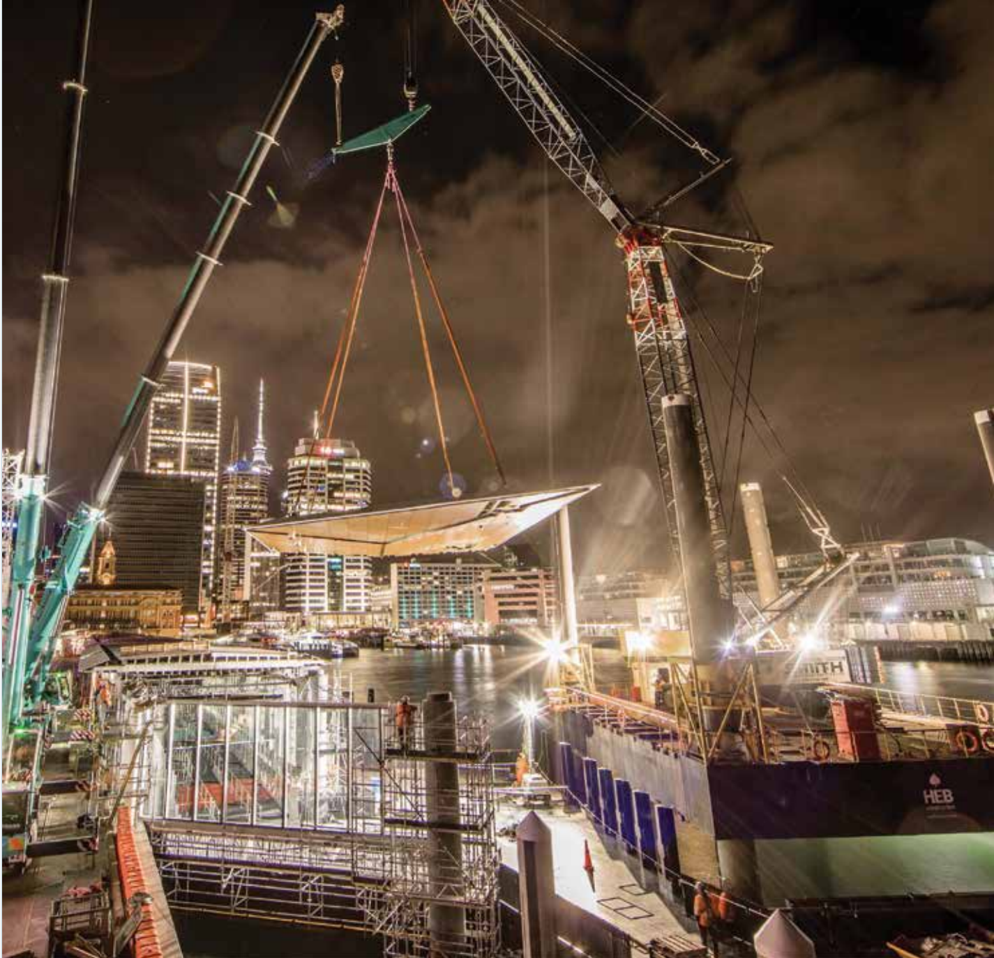
The Ferry Basin redevelopment roof canopy installation project in Downtown Auckland.
