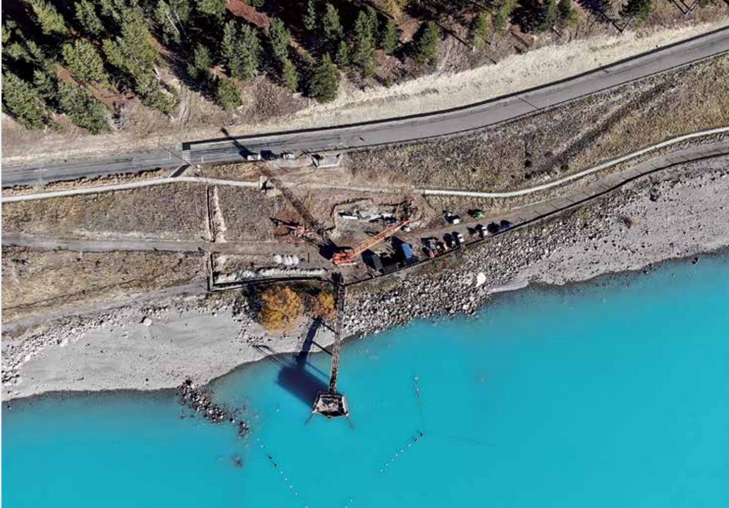
Tekapo Intake Gate Project – Downer NZ.
