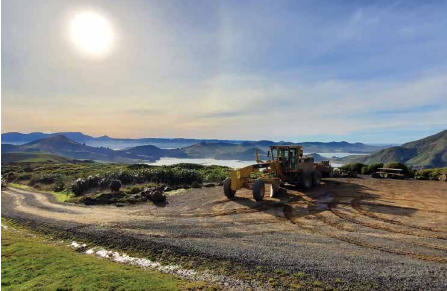
Grader clearing carpark, Dunedin – Fulton Hogan.
