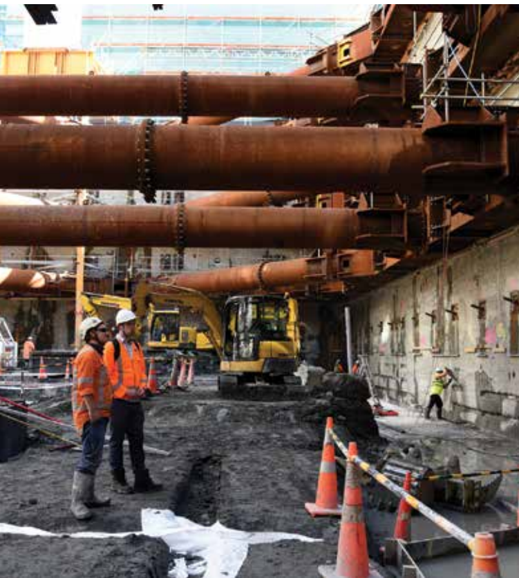
Seascope Towers Basement construction, Auckland.
