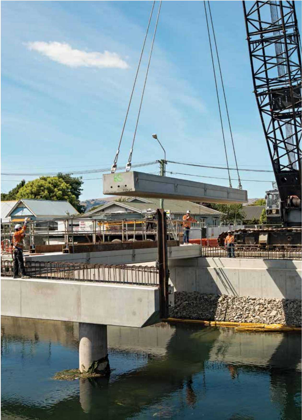
Gayhurst Bridge, part of the Stronger Christchurch Infrastructure Rebuild.
