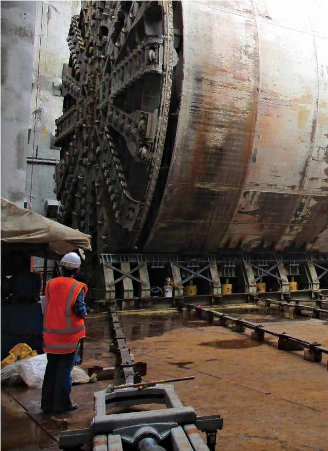
'Alice' the tunnel boring machine, Waterview Connection, Auckland.
