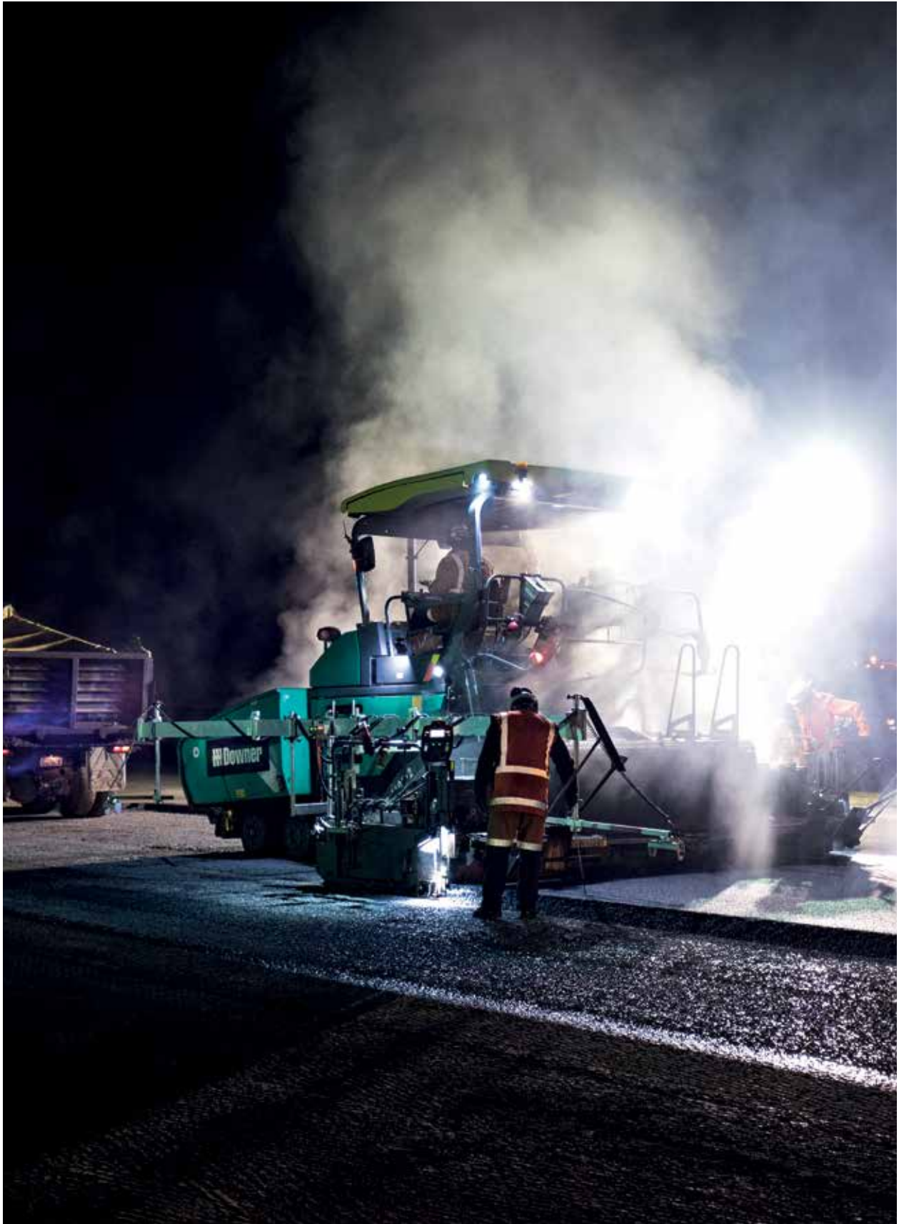
Night resealing of Gisborne airport runway in 2015.
