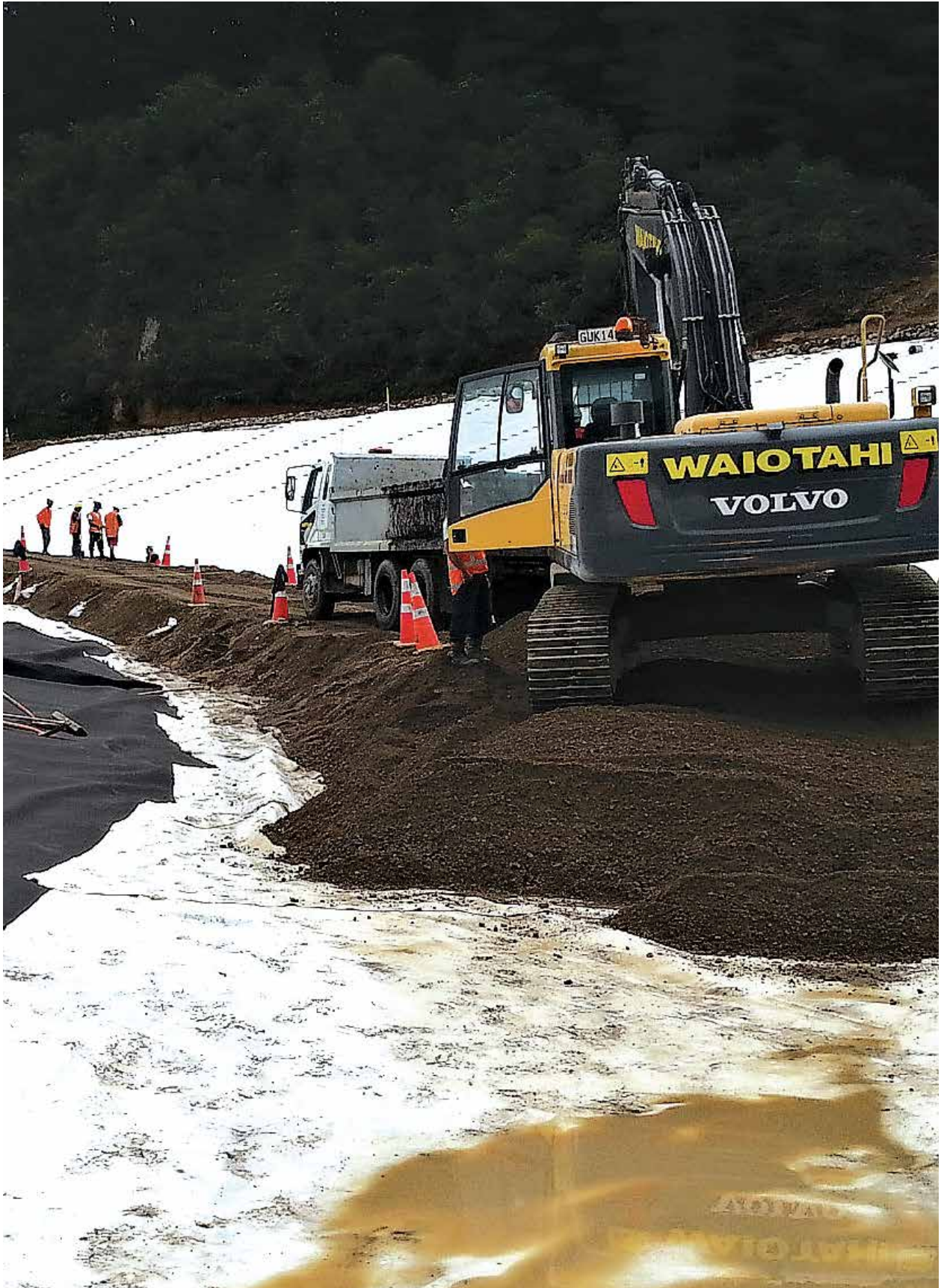
Aniwhenua Dam Head Wall Remediation works, Kaingaroa Forest, Bay of Plenty.
