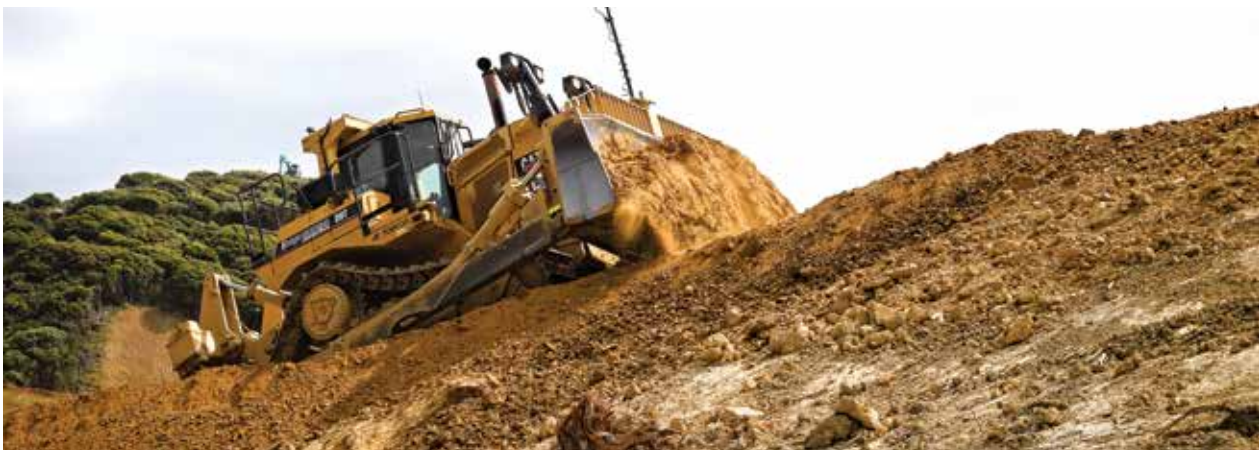
Dozer at work, Transmission Gully.
