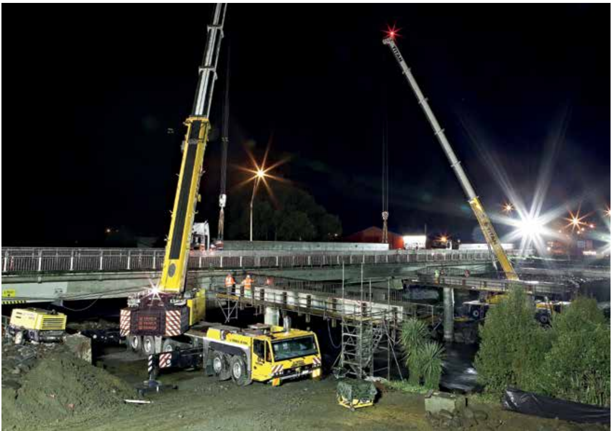
State Highway 3, Vickers to City Upgrade, Taranaki.
