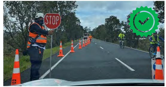
Example of a stop/go operation having a specific phase for cyclists – separating their safe travel in a single lane environment by time (from vehicles). Image Credit xlii: Betty Mitrova.
