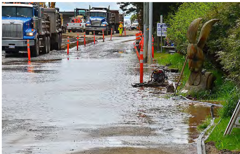
Water can pool in various places, especially in construction environments where the topography has changed. This photo is an extreme version, but even a blocked drain due to construction debris can have an impact on the safety of vulnerable road users in a worksite. Image Credit lxviii: Campbell River Mirror.
