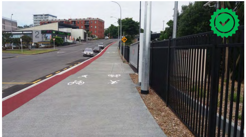
An example of a permanent shared path using pavement marking to provide directional guidance (keep left). Image Credit xviii: Waka Kotahi [70]
