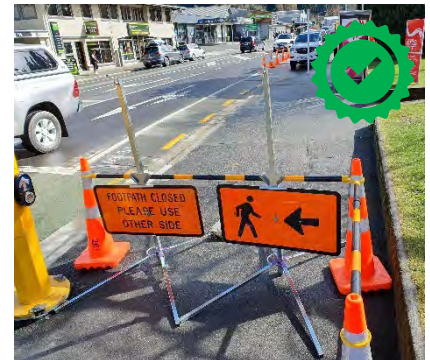
Footpath closure at signalised crossing to allow safe controlled crossing of the road for footpath users. Image Credit xlviii: Danny Wood.
