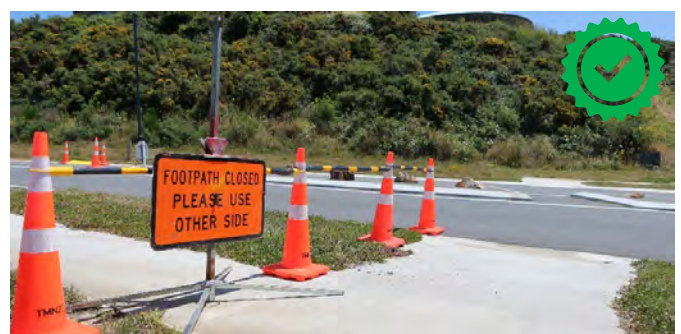
Example of footpath closure (suing other side) utilising an existing pedestrian refuge. Image Credit xlix: Danny Wood.
