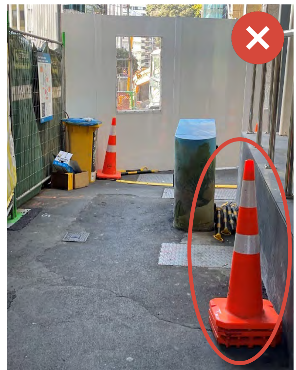
Equipment left in or adjacent to pedestrian routes that is unused only serves to add obstacles or hazards to users. Image Credit Ivii: Betty Mitrova.
