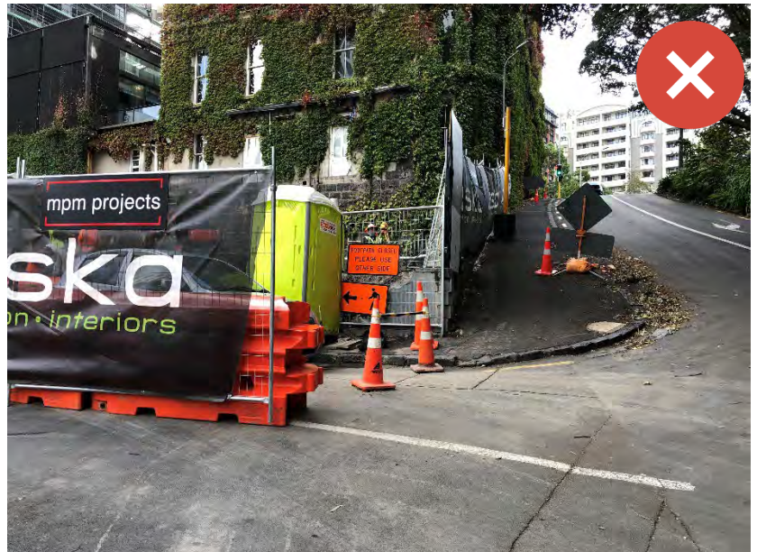
When the access gate is open on this site, the pedestrian signage directs users to walk into the site entry point. Image Credit liv: Parallaxx.
