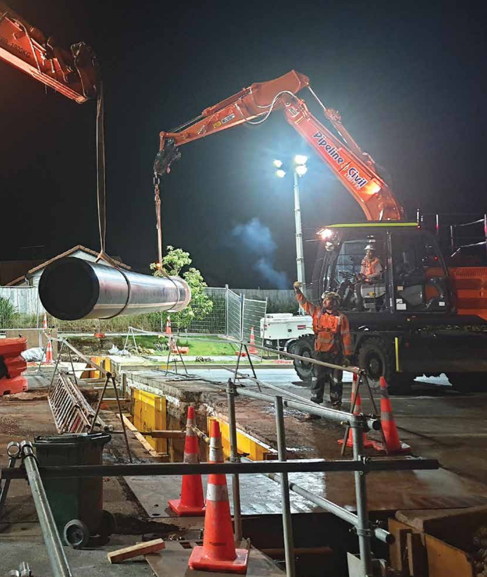
Northern Interceptor night shift crew putting a pipe in its place.
