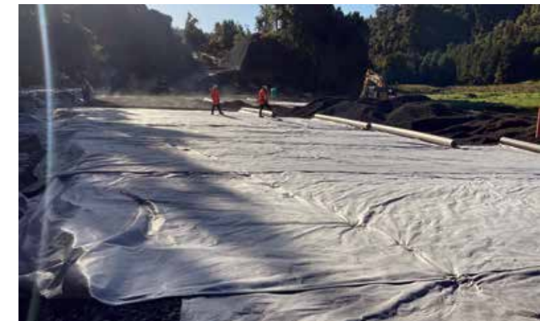
The Mount Messenger Bypass – Downer, HEB, WSP and Tonkin + Taylor
