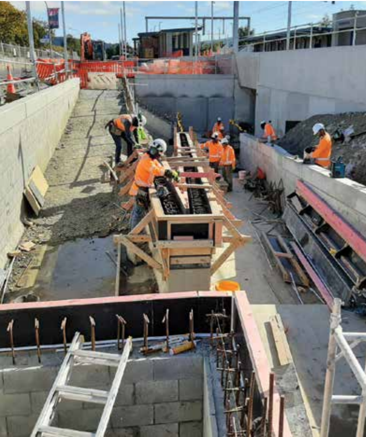
Electrification of the Trentham to Upper Hutt rail line
