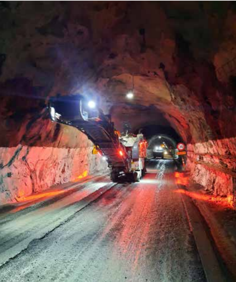
Homer Tunnel Resurfacing Works - Downer NZ
