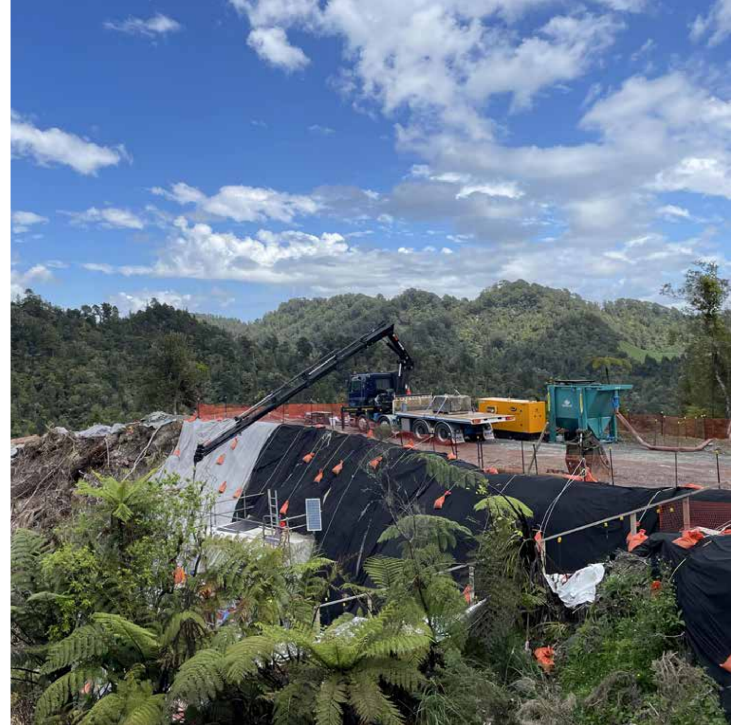
Mount Messenger Bypass tower site, looking towards the south anchors just before the installation of the tower
