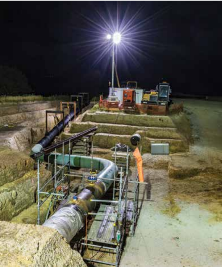
Maui Gas Pipeline – First Gas
