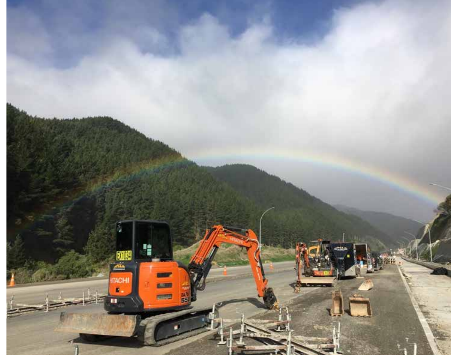
Transmission Gully Channel Drains- PCL Contracting
