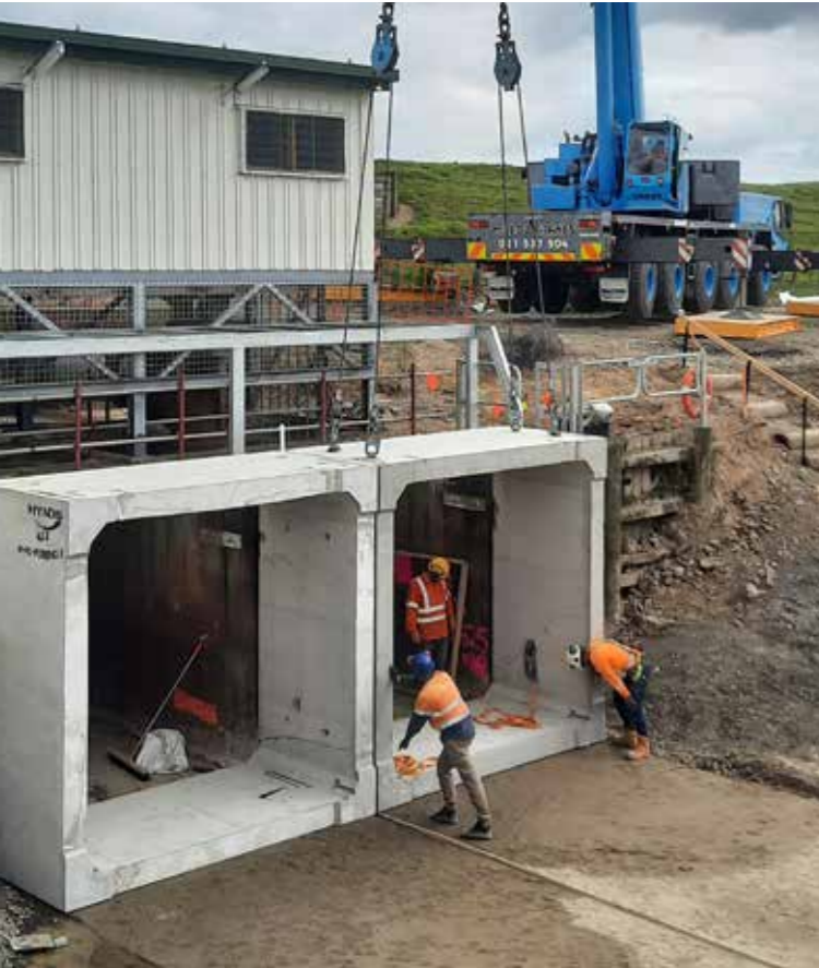
Mill Road Pump Stations No 1 & No 2 upgrade – Brian Perry Civil
