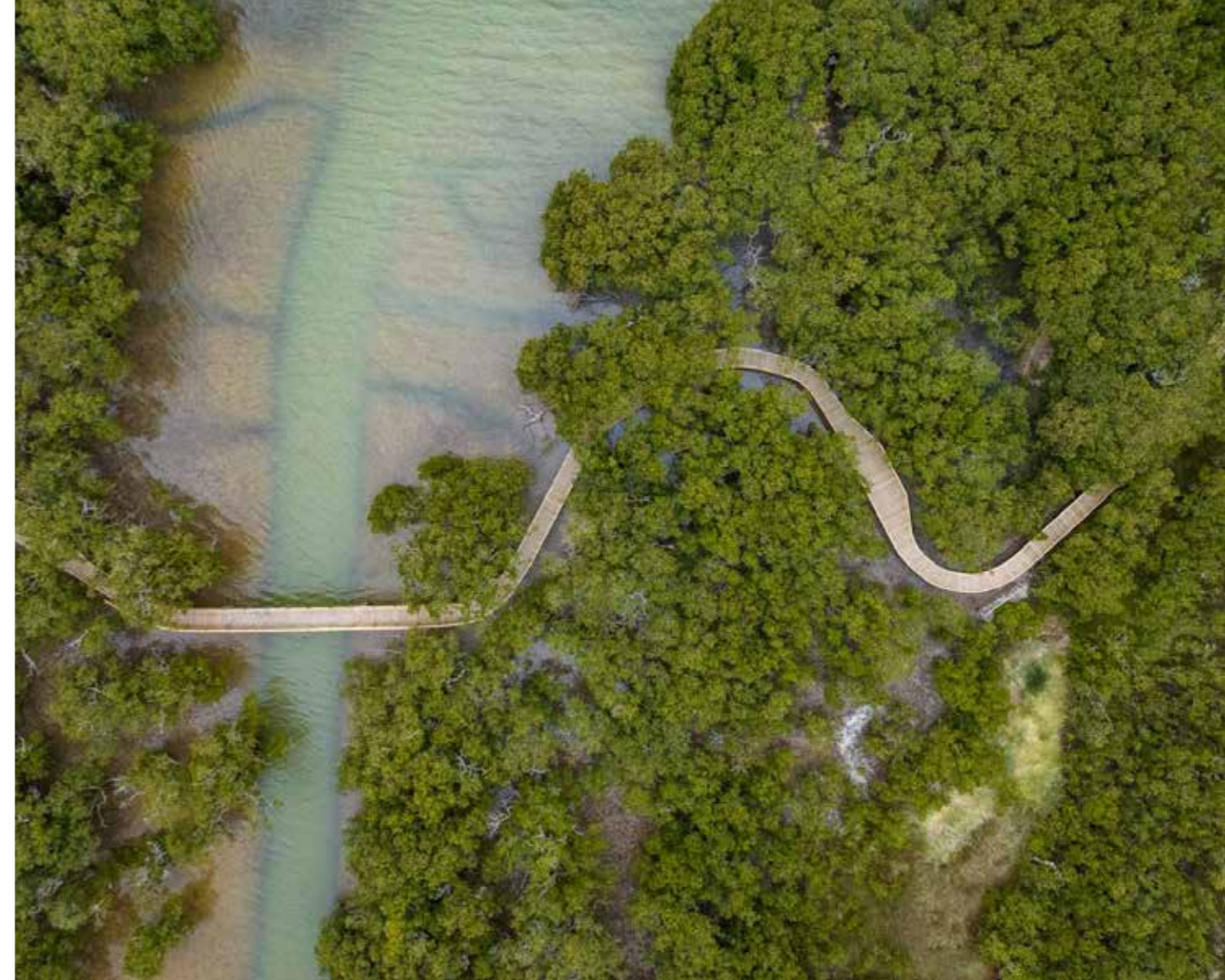
Paihia to Opuia Coastal Walkway – Stage 1 Bridge and Boardwalk Replacement – Steve Bowling Contracting
