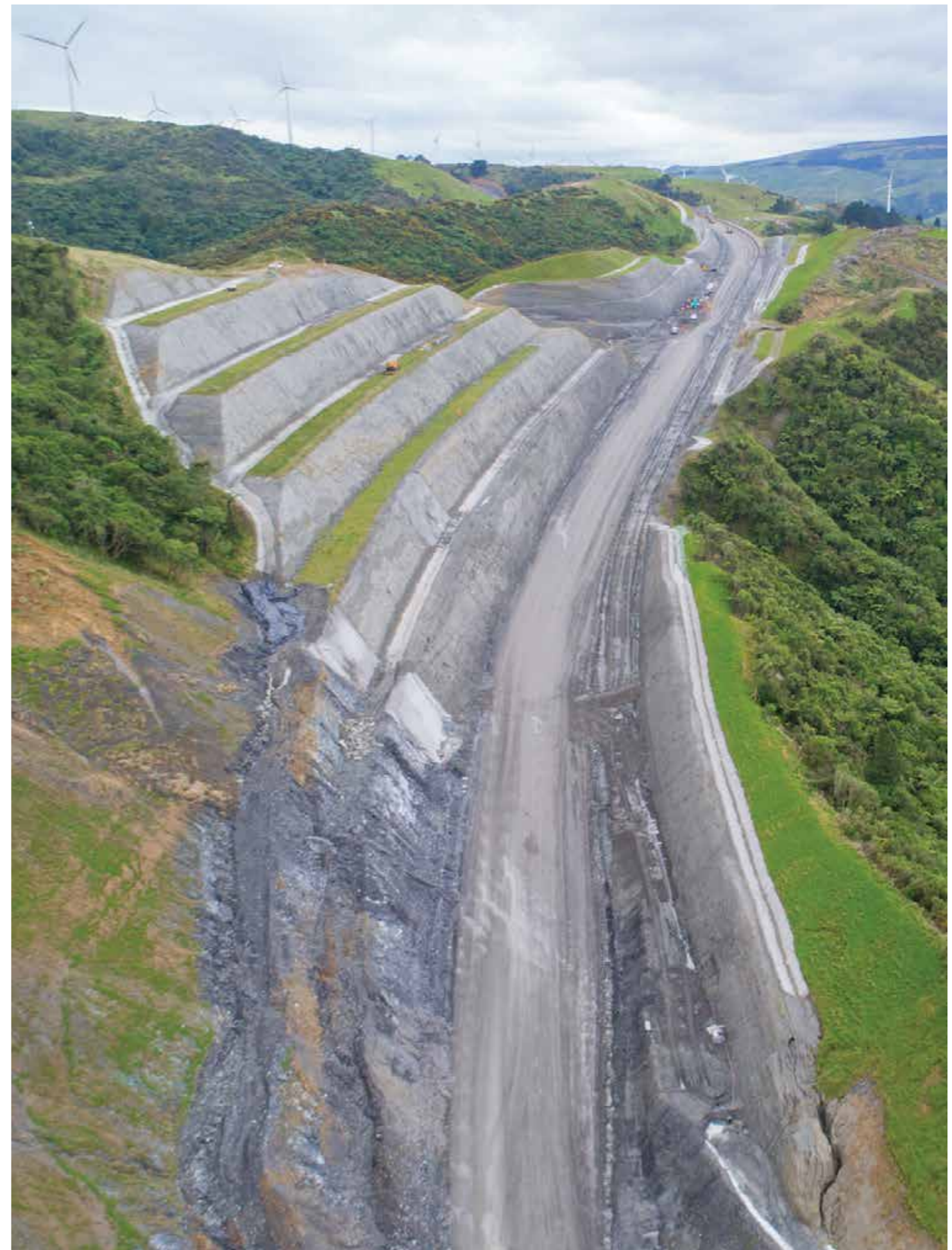
11.5 kilometre Manawatū to Tararua Highway (SH3) – HEB Construction
