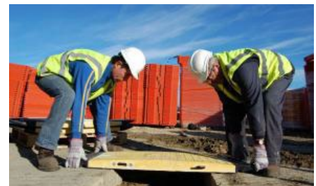
Some excavation covers can be heavy, therefore installation and removal using mechanical means is preferred. Image Credit lxxxiv: Oxford Plastics
