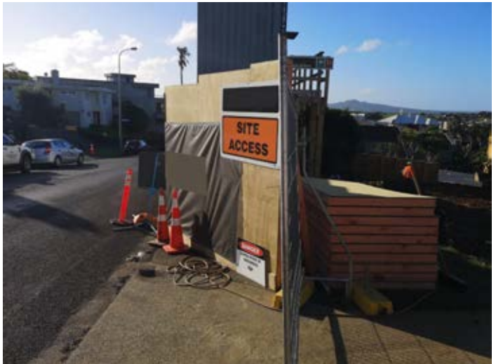
Site access and exit in this location would be very challenging. Pedestrians interacting in the same place as entering vehicles and a blind corner of hoarding close to a live traffic lane. This location would require a number of control measures to ensure the safety of site entry and exit activity. Image Credit Ixiii: Parallax.
