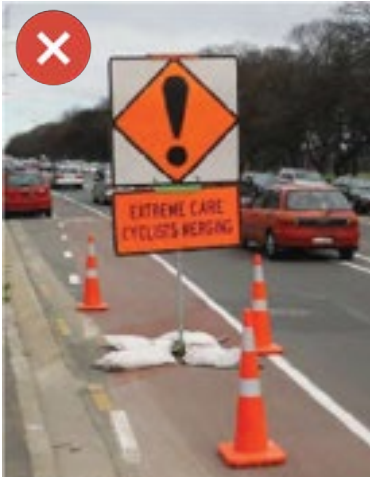
Advanced warning can help inform drivers and VRUs about upcoming hazards. Make sure not to place signs where they become a hazard themselves. Image Credit Ixxiv: Christchurch City Council.
