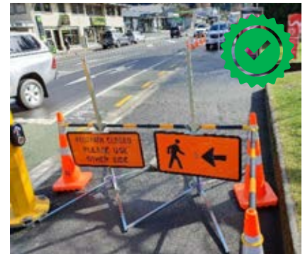
Footpath closure at signalised crossing to allow safe controlled crossing of the road for footpath users. Image Credit xlvi: Danny Wood.
