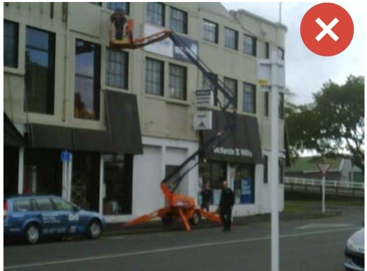
The person working on the elevated work platform has tools and materials that may fall onto the walkway below. The EWP is blocking the footpath. Image Credit xxx: Peter Graham.
