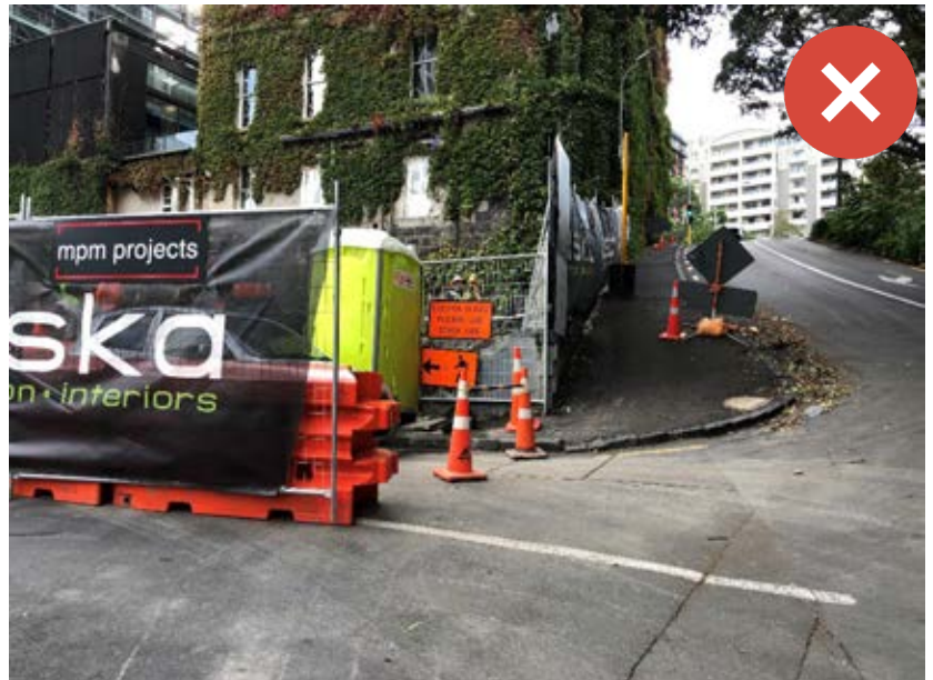
When the access gate is open on this site, the pedestrian signage directs users to walk into the site entry point. Image Credit liv: Parallaxx.
