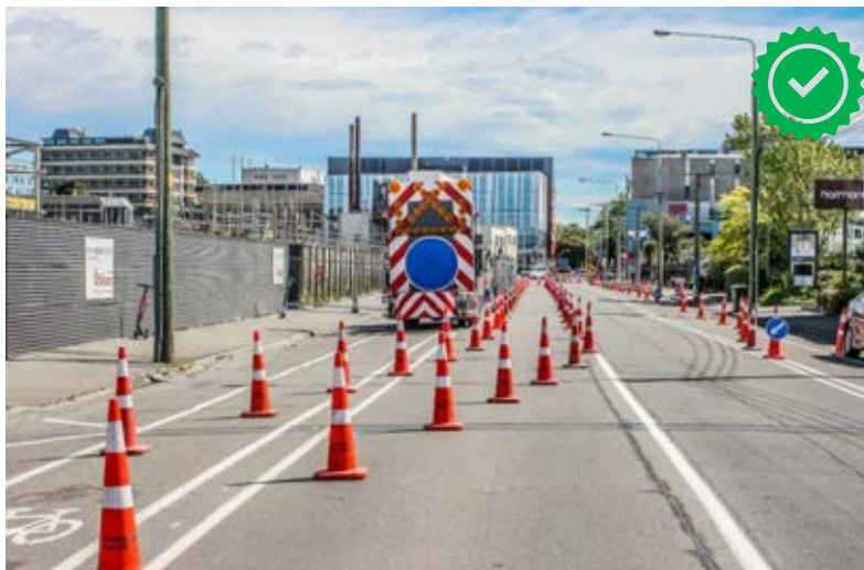
This example shows a clear and well aligned temporary cycle lane diversion. One improvement would be adding a method to prevent cyclists riding through the cones (especially at the diversion location). Image Credit xlv: Whites Traffic Management.
