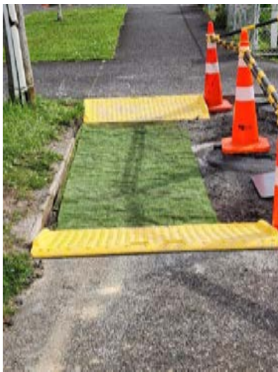
Kerb ramps can be useful for changes in elevation in other places, not just kerbs. Image Credit xc: Steve Murphy.
