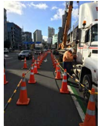
A well-formed temporary walkway is well marked, straight and clear, and separated from other hazards like work activity and live traffic. Image Credit cv: Parallaxx.
