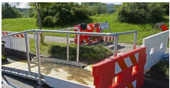
Pedestrian kerb ramps come in many forms, including more robustly constructed types such as this one. Kerb ramps that are fit for purpose based on the situation, duration, and risk for the site should be selected. Image Credit xci: Oregon Department of Transportation.
