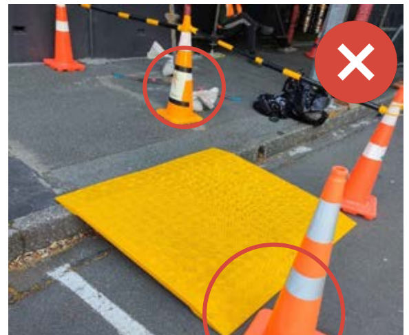
The use of paper taped to a cone has meant the sign has deteriorated and hardly visible. The cone makes the ramp narrower which is particularly problematic for people using a wheelchair. Image Credit Iv: Betty Mitrova.
