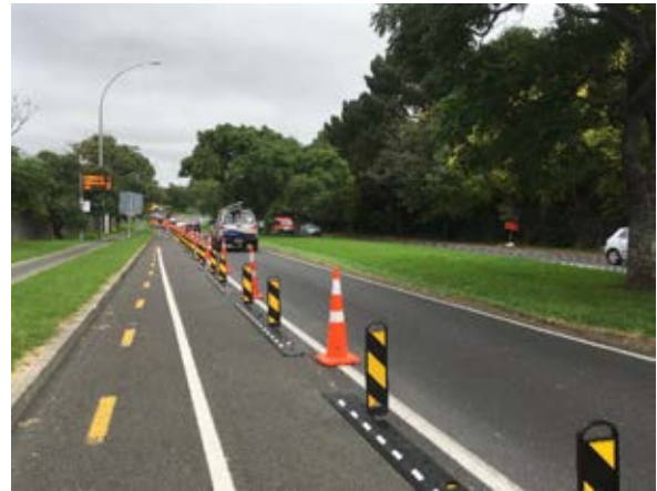
Delineation between cycle paths and live traffic is vital for ensuring safe separation. Image Credit to: Bike Auckland.
