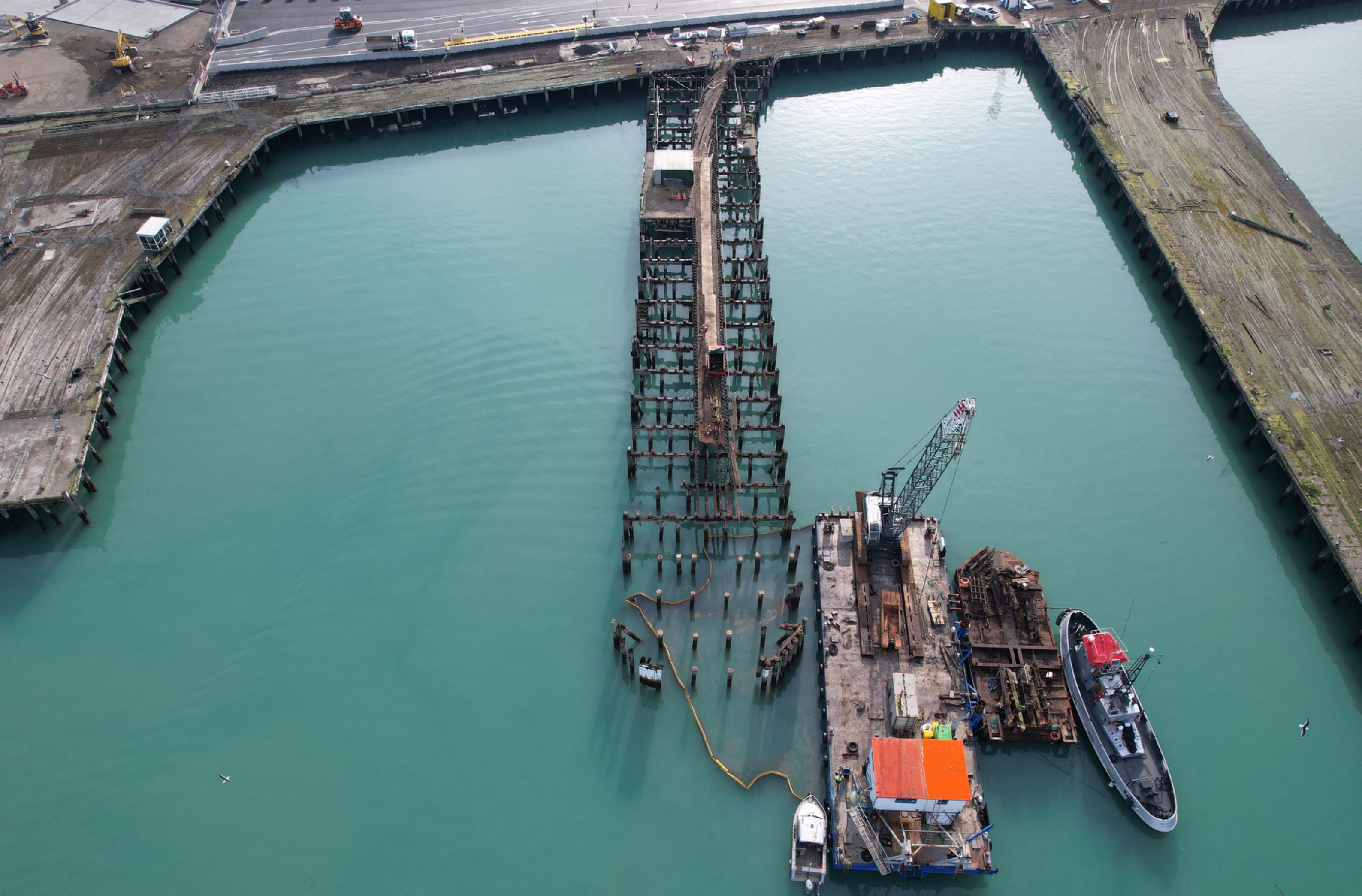
ALANA FROM SMITH CRANE AND CONSTRUCTION, AT LYTTLETON PORT, CHRISTCHURCH - SMITH CRANE AND CONSTRUCTION'S CIVIL TEAM HITS THE WATER TO DISASSEMBLE JETTY
