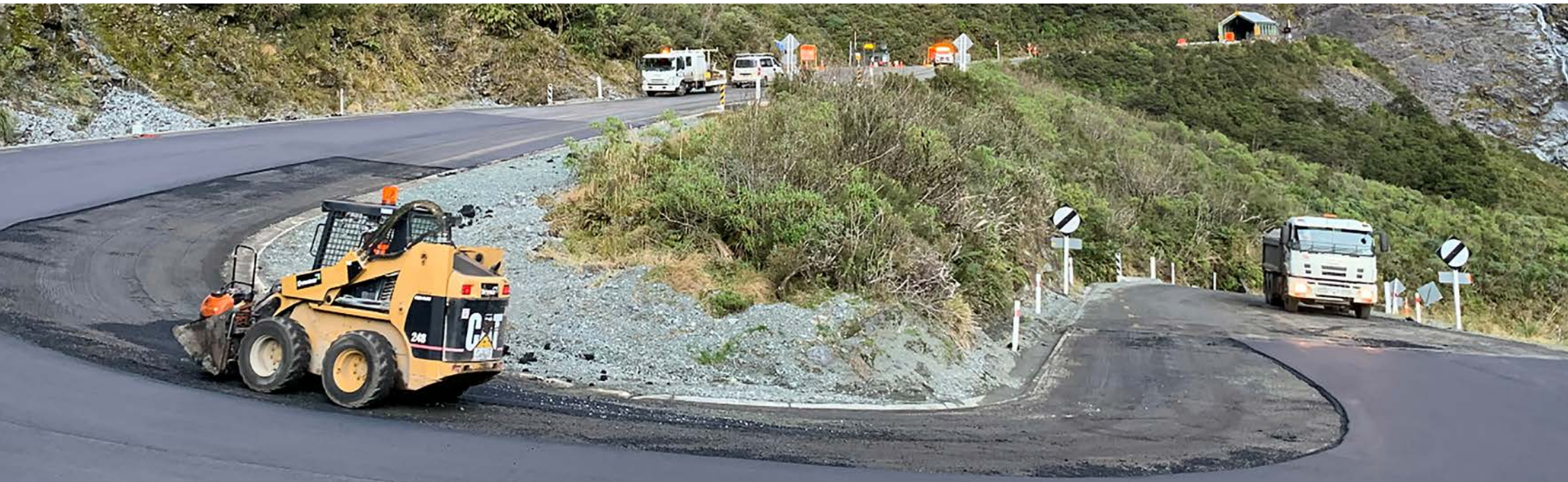
Homer Tunnel resurfacing works Photo provided by Downer NZ
