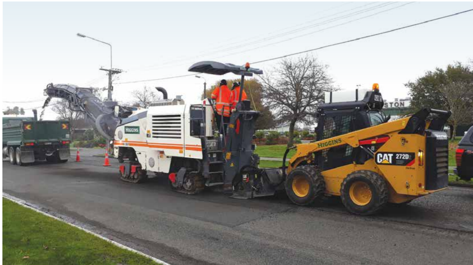
Higgins Contractors at work in Southland.
