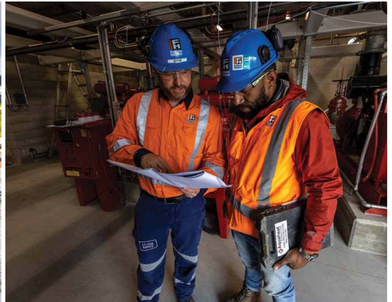
The Ohakea RNZAF Base fire station pump house.
