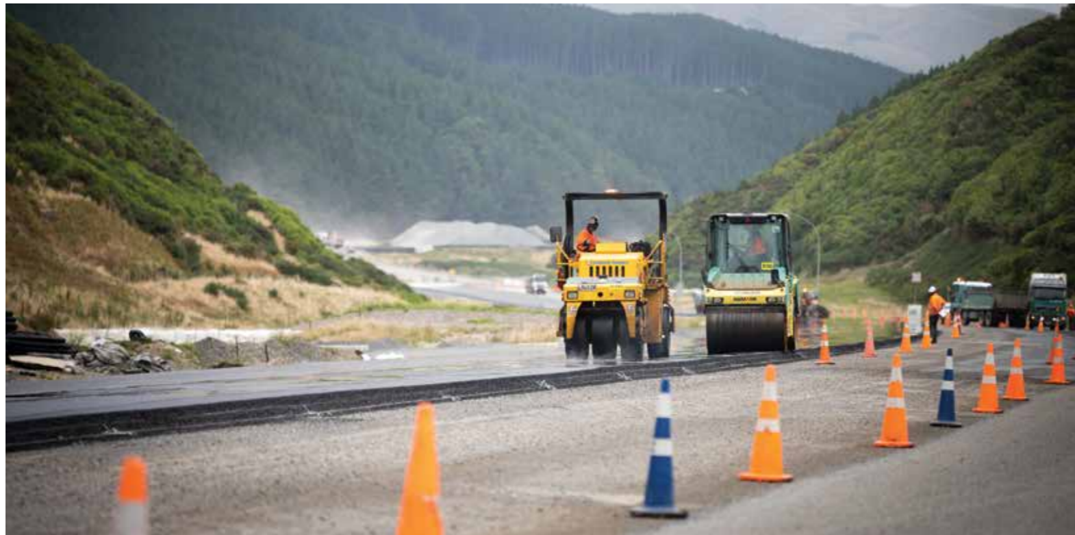
Rollers compact the newly laid deep lift asphalt along a section of the Transmission Gully motorway.
