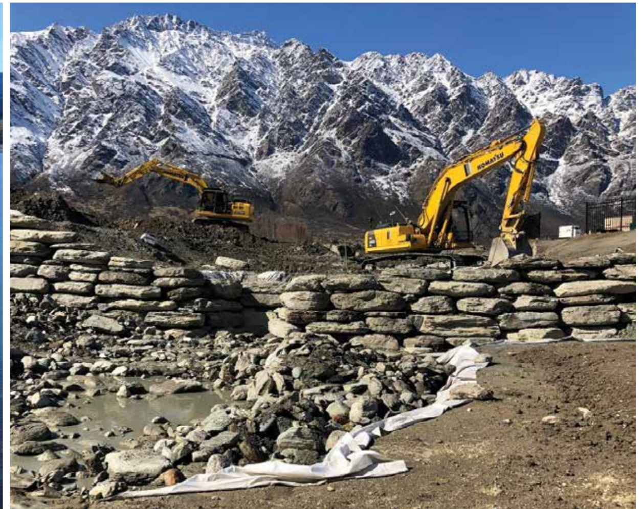
Base Contracting 2003 Ltd in action on a spectacular Queenstown day.
