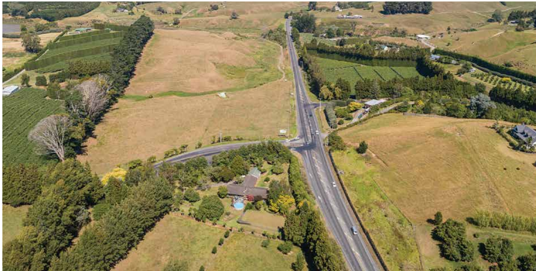
State Highway 2, Omokoroa Road intersection January 2021.
