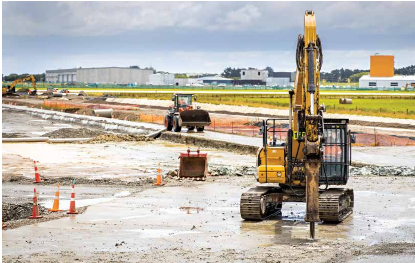
Demolition of the old taxiway and earthworks at RNZAF Ohakea.
