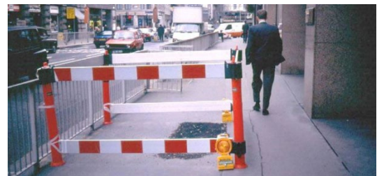
This image from the U.S. shows the concept of a detectible edge – illustrating a limitation of using cone bars in TTM. Image Credit Ixxvii: Dan Burden.
