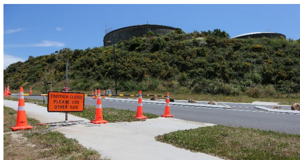
When selecting crossing points, using existing permanent infrastructure (including median refuges) is preferred. Image Credit xcvi: Danny Wood.
