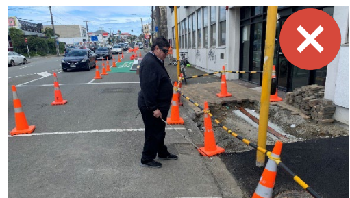
A shortfall of cone bars is they have no detectible edge for cane users. Image Credit Ixxviii: Waka Kotahi.
