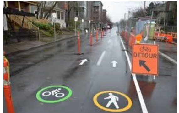
Markings can be used to help give clear guidance of separation of users. Using colours is also valuable for those with visual impairments. Image Credit xcii: Bike Portland.
