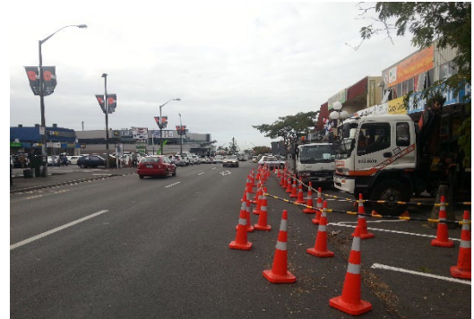
Delineation serves to channel different types of road users with a primary purpose of being visible. Image Credit Ixxix: Parallax.
