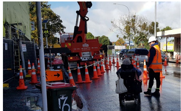
Having staff on hand to escort and assist those with disabilities is a very effective way to ensure sites are able to be navigated safely by even the most disadvantaged of users. Image Credit lxxx1: Parallax.
