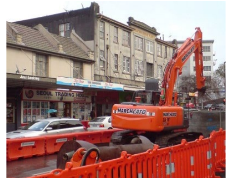
Fencing is particularly important on longer-term worksites, and where heavy machinery is used. Image Credit lxxxvi: Wikimedia Commons.
