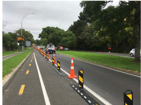
Delineation between cycle paths and live traffic is vital for ensuring safe separation. Image Credit ci: Bike Auckland.
