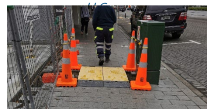
Covers placed on footpaths should be bright and flanked by devices that show clearly the safe path for VRUs. Image Credit lxxxv: Carina Duke.
