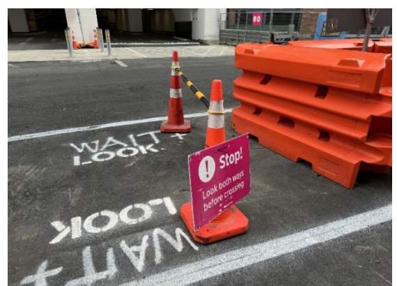
In many cases, VRUs look down – so marking can be a valuable way to provide guidance that supports signs and places information exactly where they are looking. Image Credit xciii: Parallax.
