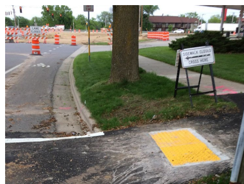
Tactile Ground Surface Indicators are an important measure for the safety of pedestrians, even at temporary crossing points. They should be considered in accordance with best local practice. Image Credit c: UW-TOPS Lab.
