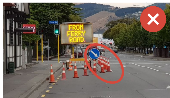
When placing delineation next to traffic lanes – don't put it right up to the lane line/edgeline. Leave space for a small 'shoulder space' for safe cycling (at least 0.5m). Image Credit Ixxix: Glen Koorey.
