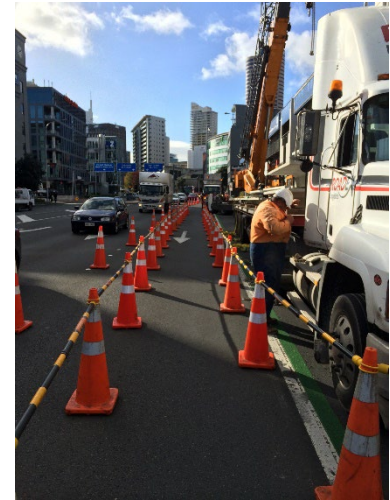
A well-formed temporary walkway is well marked, straight and clear, and separated from other hazards like work activity and live traffic. Image Credit cv: Parallax.
