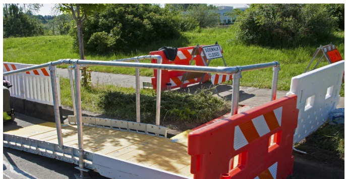
Pedestrian kerb ramps come in many forms, including more robustly constructed types such as this one. Kerb ramps that are fit for purpose based on the situation, duration, and risk for the site should be selected. Image Credit xci: Oregon Department of Transportation.
